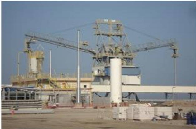
Ship unloader and quay conveyor
