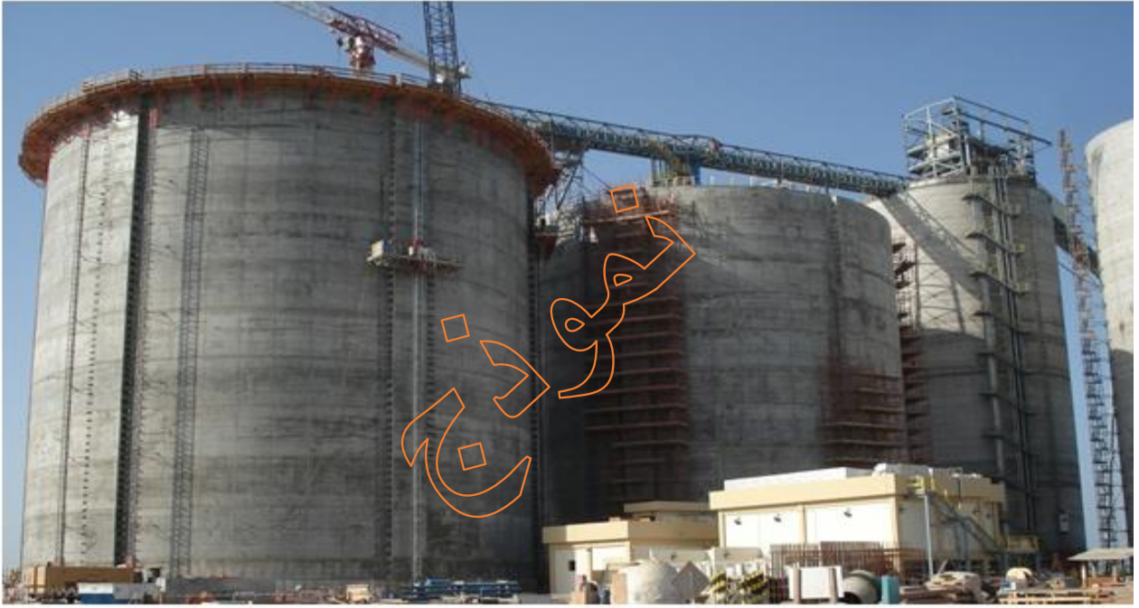
Installation of material handling system to alumina conveyors
