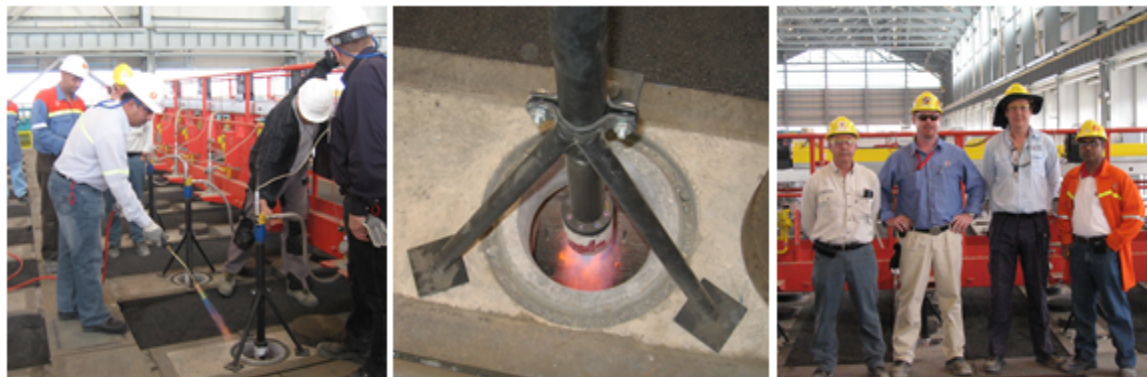
Dry out of the Anode Bake Furnace commenced in March
