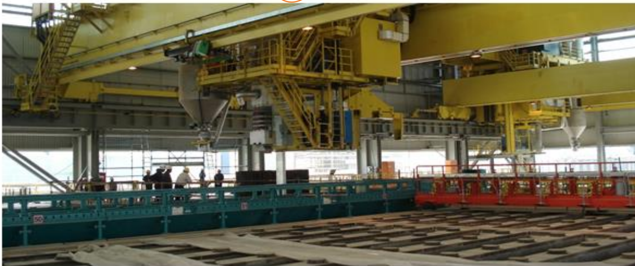
ABF tub filling in preparation to start the dry-out fire
