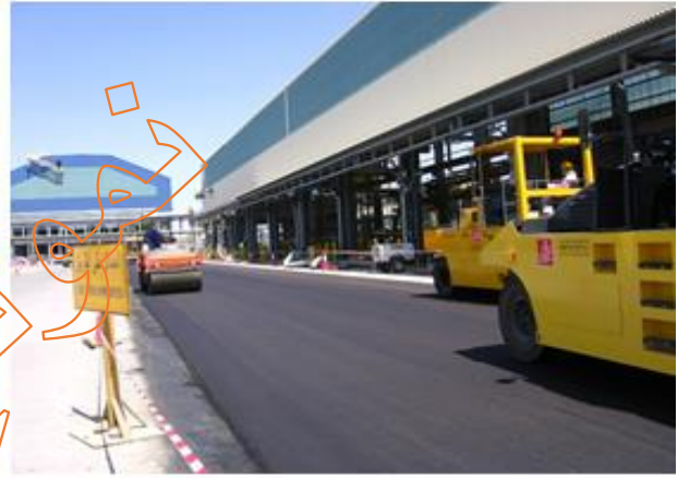
Asphalting outside the Crucible Cleaning Shop
