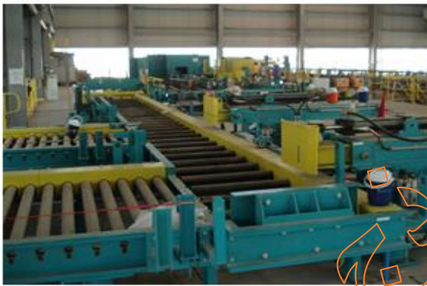
Pre-Commissioning of the Anode Handling system inside the ABF
